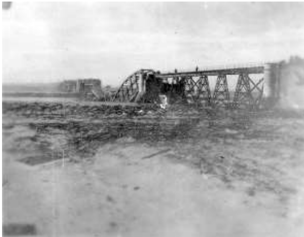
Destroyed Mook Railway bridge over the River Maas
